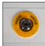
Tomas Gases medicinales Medical gases outlets
