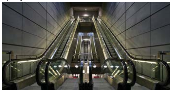
Copenhagen Metro – 370 unit. FCU
