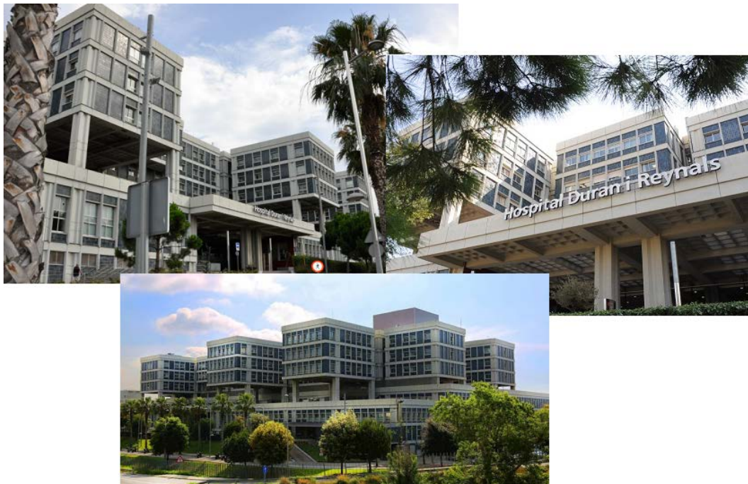
Hospital Durant i Reynals ICO – 730 unit. FCU
